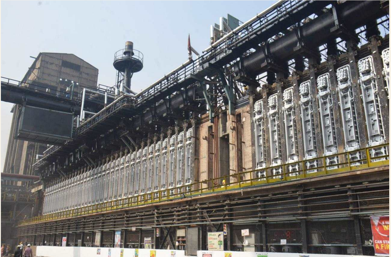
A coke oven battery at an Indian steel plant.
